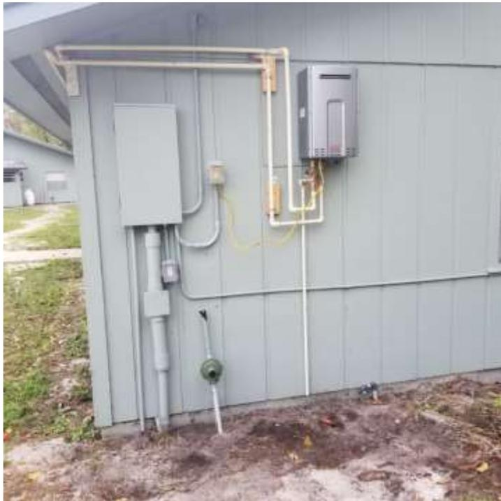
The original propane lines and regulators were no longer up to current code. We ran new lines and regulators to the original buildings. Then, the aging water heaters flunked the leak test. So, we replaced them with tankless systems (like the new cabins). This also put all of the propane on the outside of the buildings.
